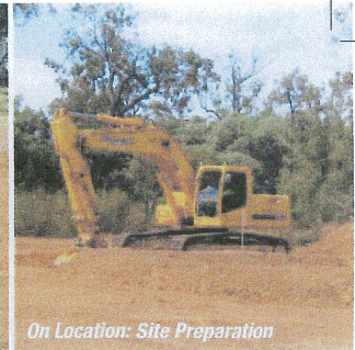
On Location: Site Preparation
